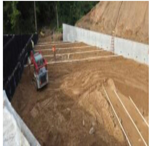
dead man footing for bridge
