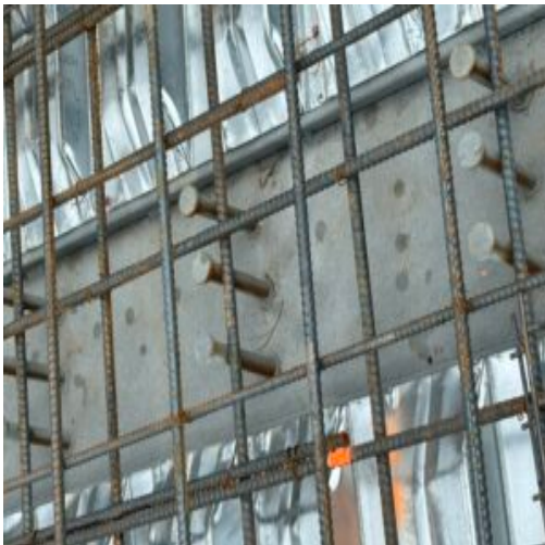
Observation of reinforcing steel being installed at bridge panels
