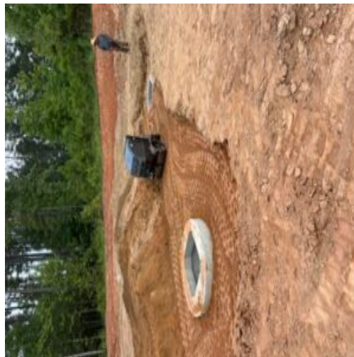
Backfill and compacting efforts at 18" rcp storm lines between Y6 & Y6.1 and 2.1 & 3.1 at unit 4 parkway phase 2
