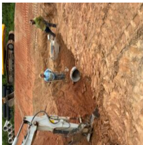
Backfill and compacting efforts at 18" rcp storm lines between Y6 & Y6.1 and 2.1 & 3.1 at unit 4 parkway phase 2
