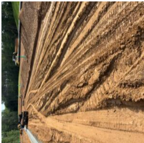
Sub grades observe at unit 3 phase 13 roadway which will require repair
