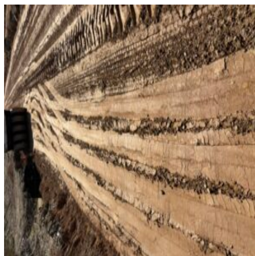
Placing sub base stone over existing sub grade
