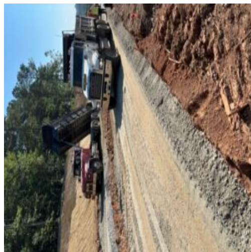
Placing sub base stone over existing sub grade
