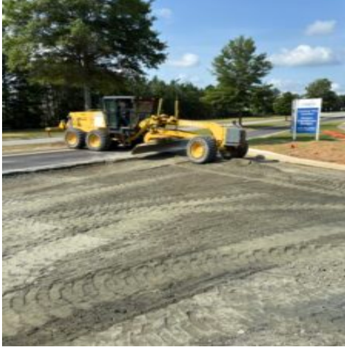
Fine grading subbase
