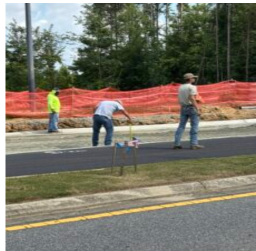
String line for depth check
