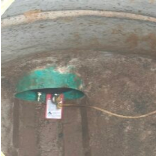
Sanitary sewer line air test Seven Hills 13
