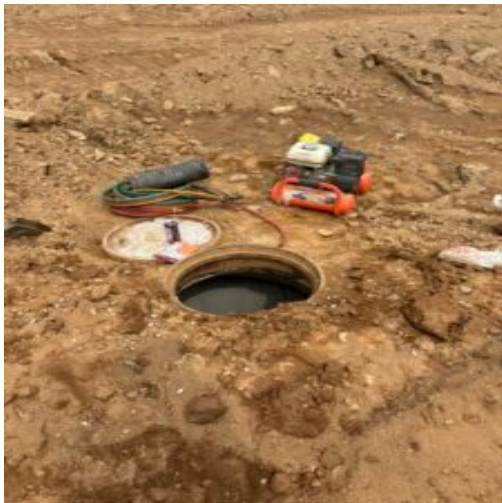
Sanitary sewer line air test Seven Hills 13
