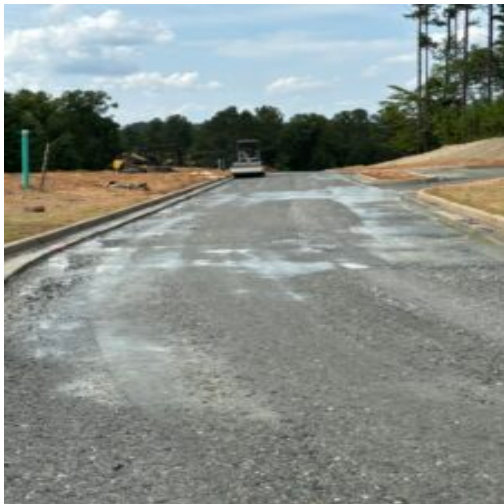
Subbase prep. at decel. lane and roadway
