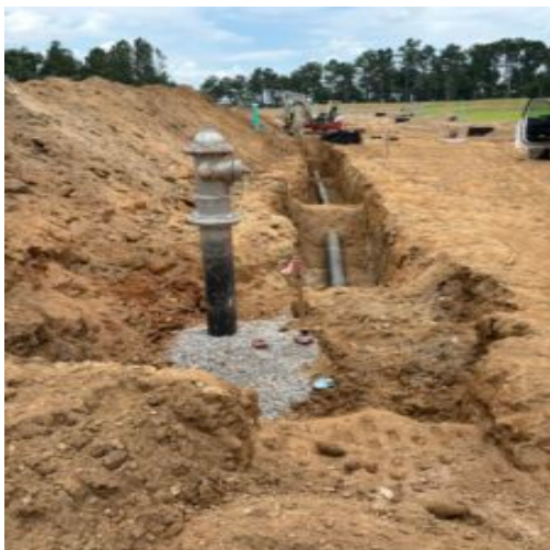
8" ductile iron water line installation unit 4 phase 2
