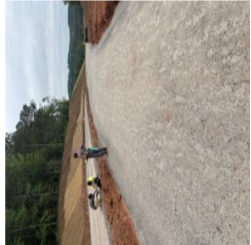
Paving contractor installing grade stakes at Nature Walk
