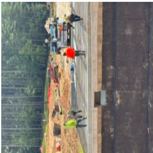
Placing re steel at bridge floor slab
