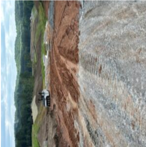
Saturated sub grade conditions at Nature Walk Pkwy.
