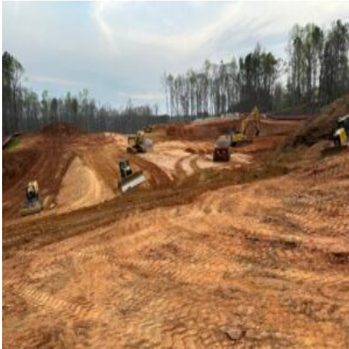
section worked at entrance
