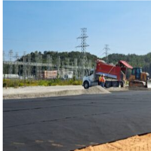
Hauling and compacting the stone on the other half of the basement
