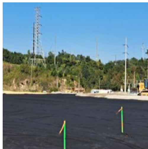
placed geo-fabric on the basement
