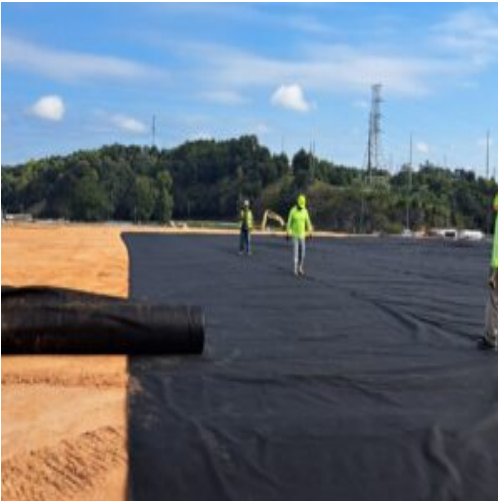
placed geo-fabric on the basement
