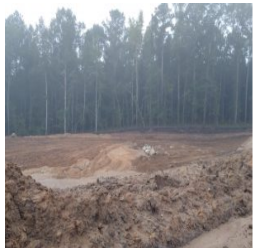
Turning up soil to dry it for future filling.
