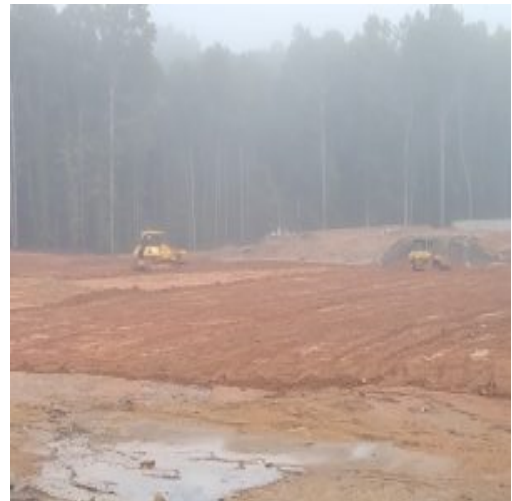
Turning up soil to dry it for future filling.
