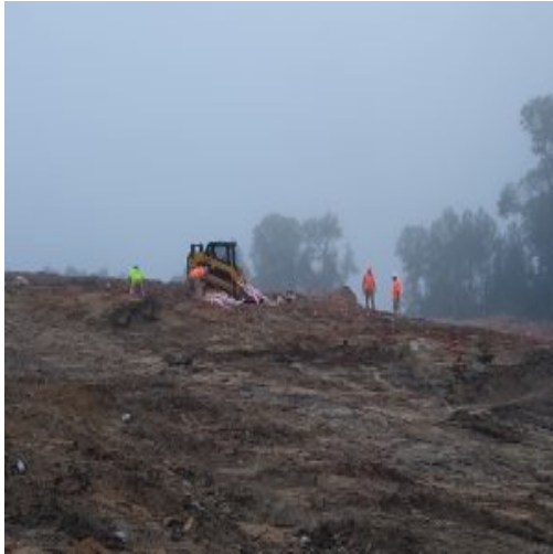
Precision blasting preparing for rock blasting.
