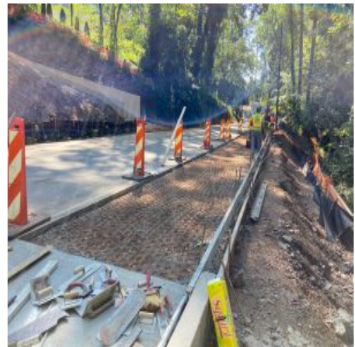
Prepared subgrade ready for concrete placement.
