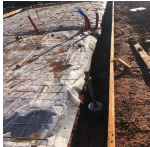
DCP testing performed
