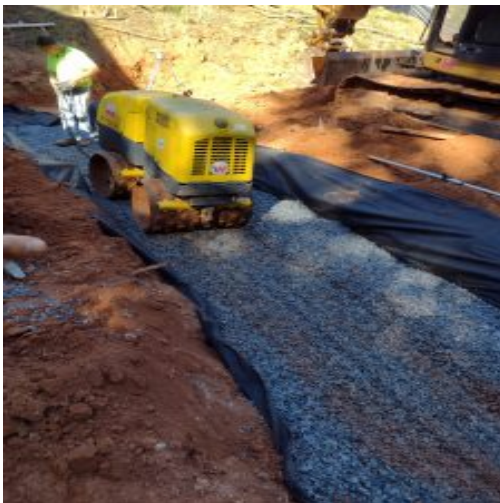
57 stone placed wrapped in fabric
