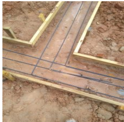
Rebar along footing on the north side
