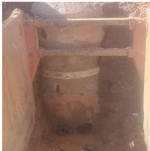
Pipe excavation on site.
