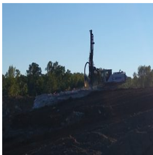
Drilling on site.
