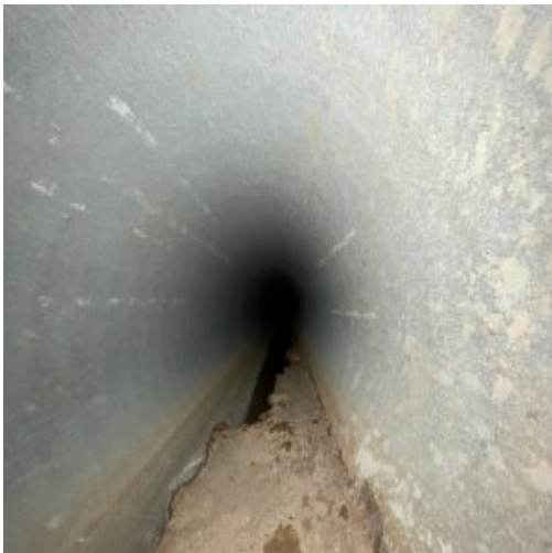
Pipe section in the north side of the structure.
