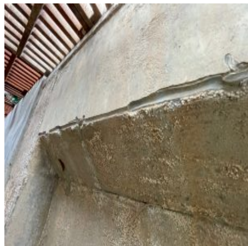
Looking at the top section closest to the grates,
