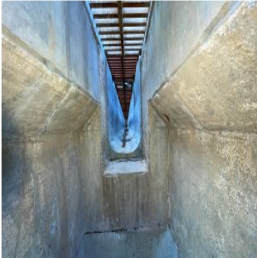
East side of the structure looking towards the trench drain.
