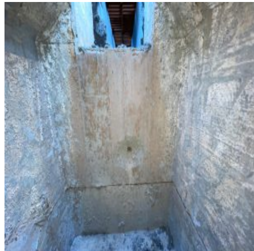
Close up view of the West side of the structure looking towards the trench drain.
