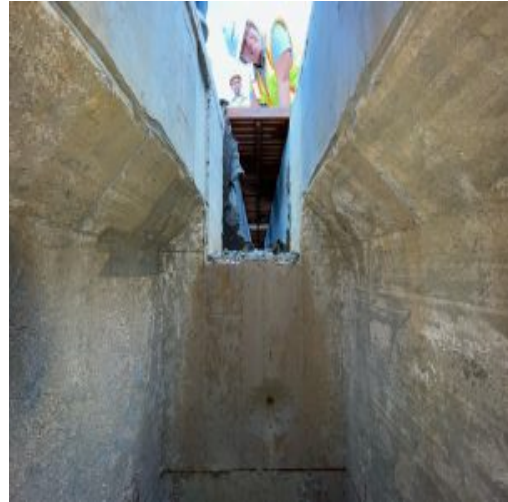
West side of the structure looking towards the trench drain.
