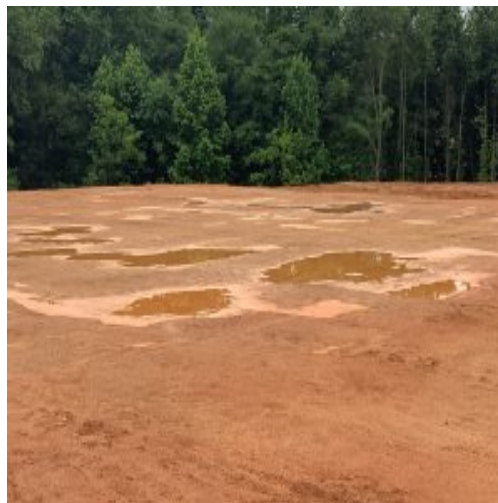
General Site Conditions
