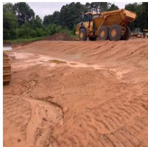
General Site Conditions
