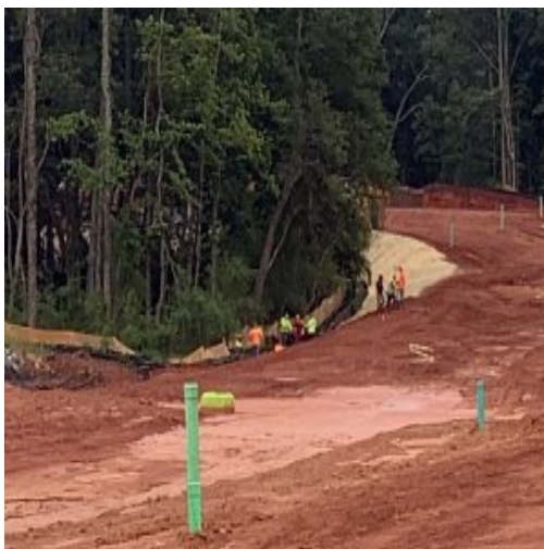
Silt Fence Relocation
