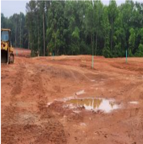
General site conditions
