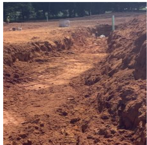
Sewer Line Excavation
