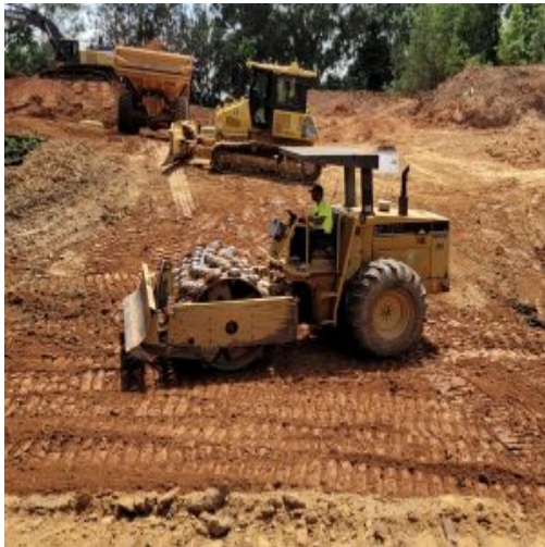
Compaction of soil bridge lift
