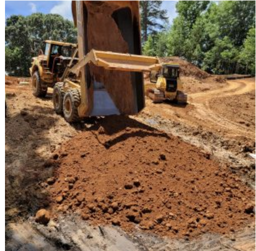
Soil Bridge uncompact fill placement
