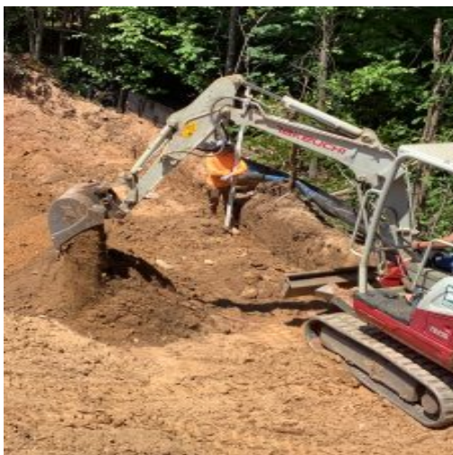
Footing Excavation Lot 228
