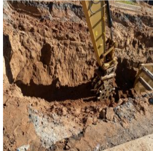
Sanitary Sewer replacement along Cannon Walk
