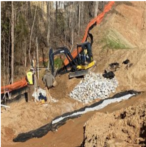
Drainage Remediation Retention Pond Outlet
