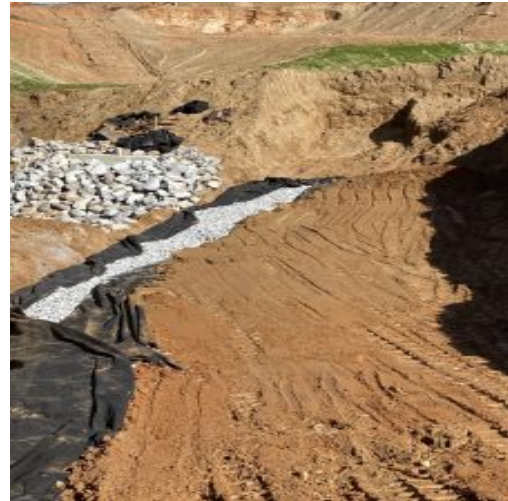
57 Stone wrapped in separation fabric - Retaining wall foundation
