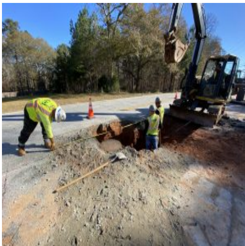
Sewer line A
