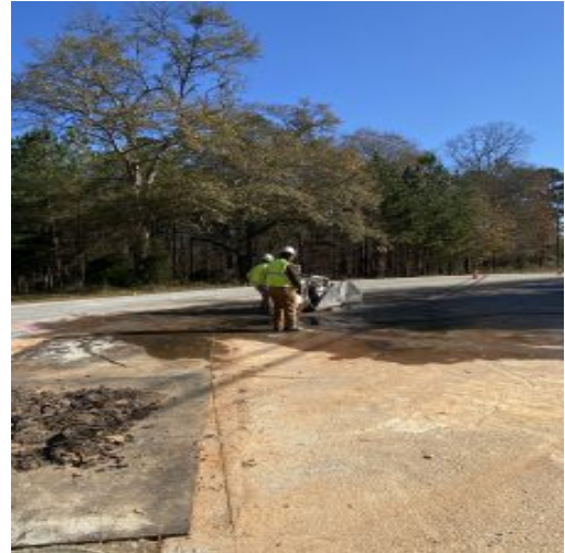
Saw Cut following Civil Plans
