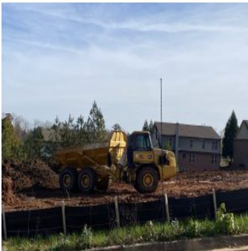
Stockpiled material Lot 18
