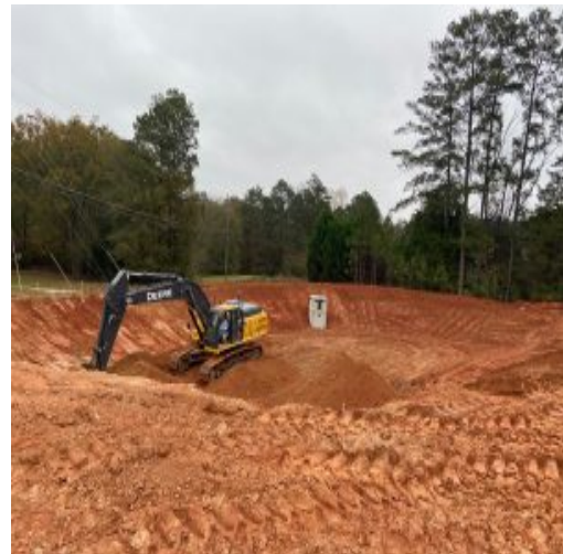
Excavation in Pond A
