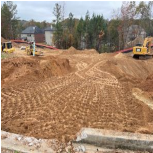
Backfill in and around lot # 9
