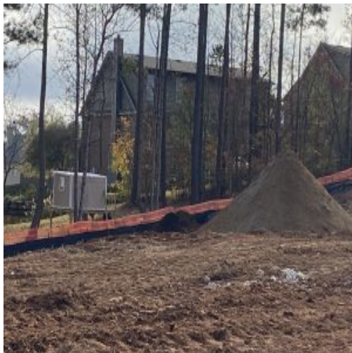
Lot 13 Trench East side of property, Not within the main building pad
