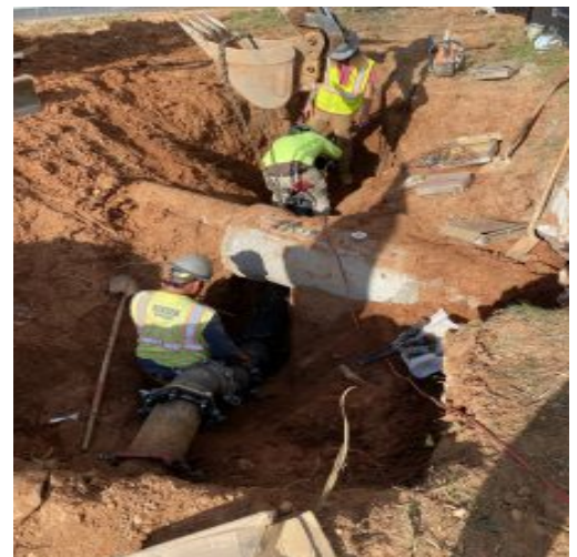
Storm Drain Line A
