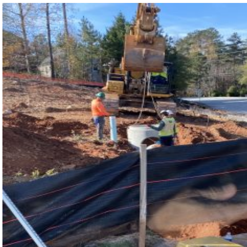
Storm Drain Pipe A ; LOT 1 North East Corner
