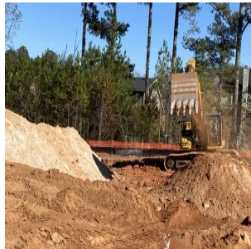
Trench area Lot 18 - 19 used for concrete rubble from various areas of site.
