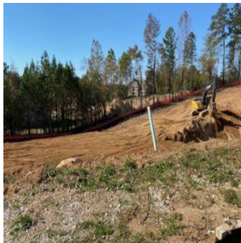
Pond B excavation ongoing
