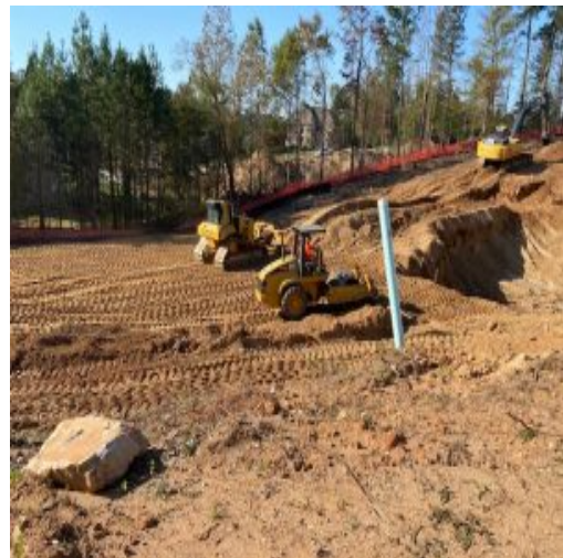
Compaction efforts during embankment placement in the vicinity of Lot # 9
