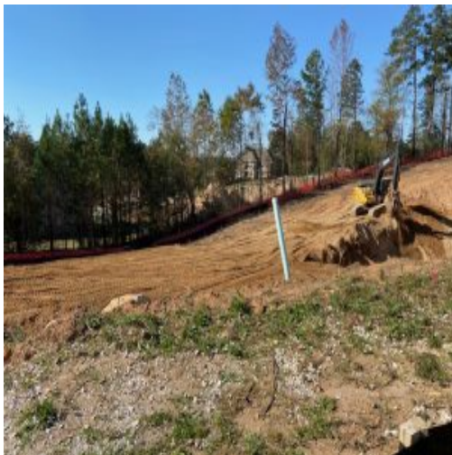
Pond B Excavation and embankment placement in the vicinity of Lot # 9
