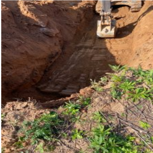
Fill placement in the vicinity of Lot 9
