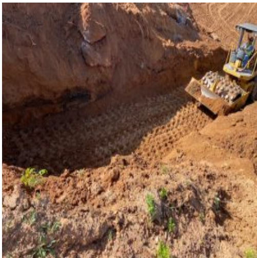
Compaction efforts using a CAT CP-433E
