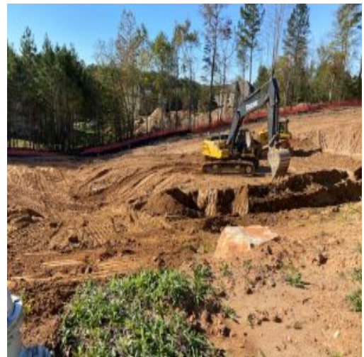
Pond B excavation
