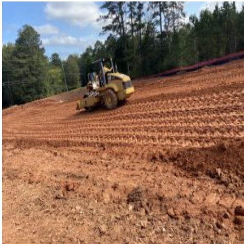
CAT CP-433E model padfoot roller performing compaction
