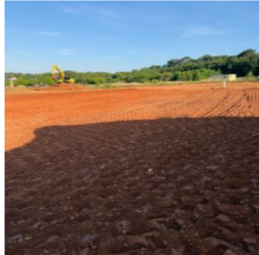
removal of top soil
