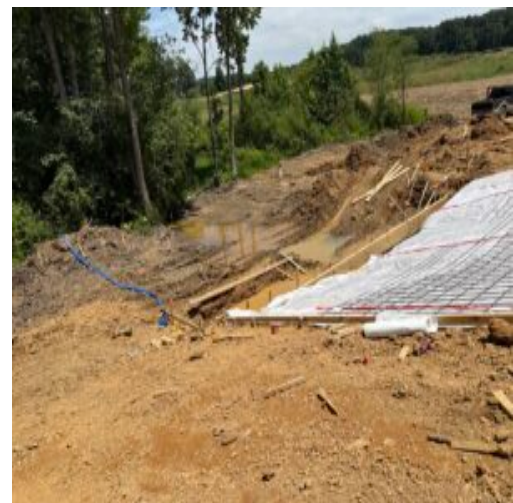
water at bottom of spillway
