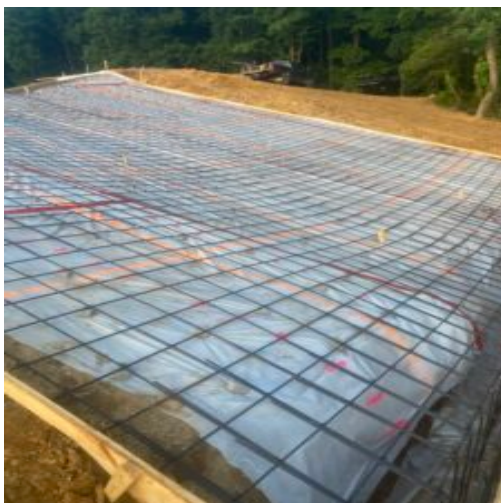
rebar placed next morning.
