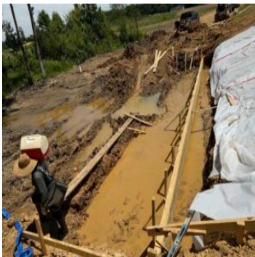
Water at bottom of spillway
