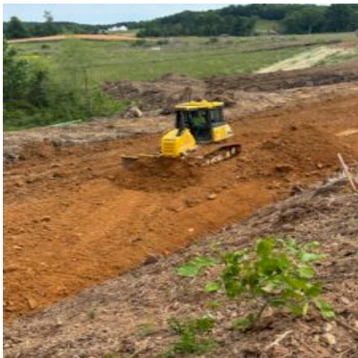
Placing fill at toe of slope
