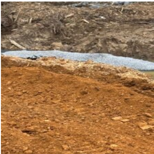
Added french drain at west end of slope
