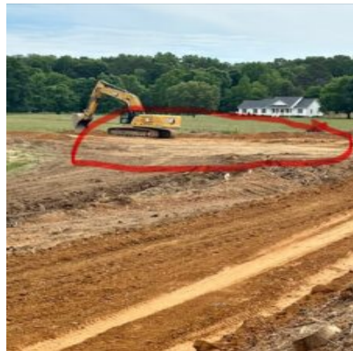
Showing area for borrowed excavated fill materials
