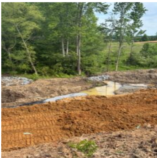
Pushing fill over french drain
