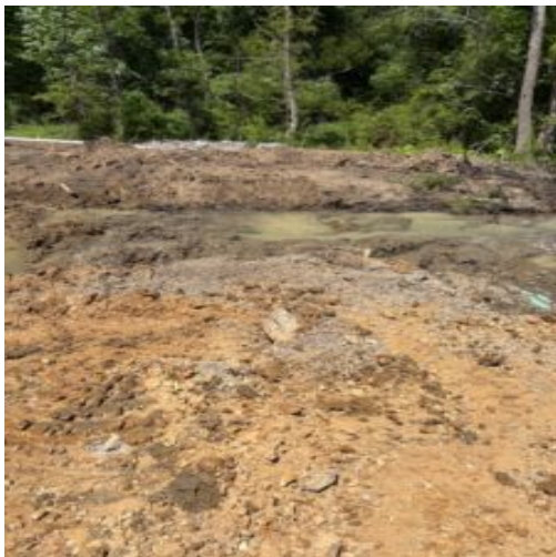
Observed saturated sub grade after excavation
