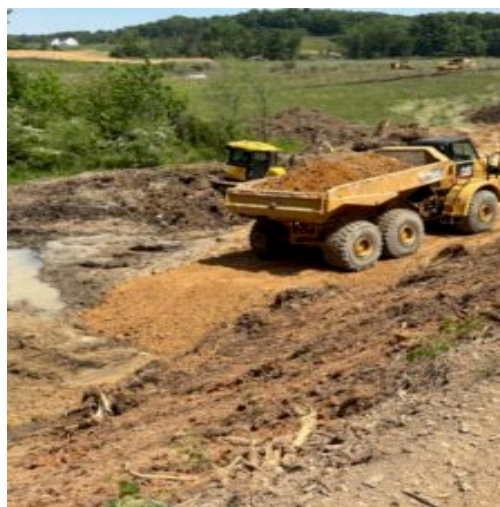
Fill placement using off road dump truck
