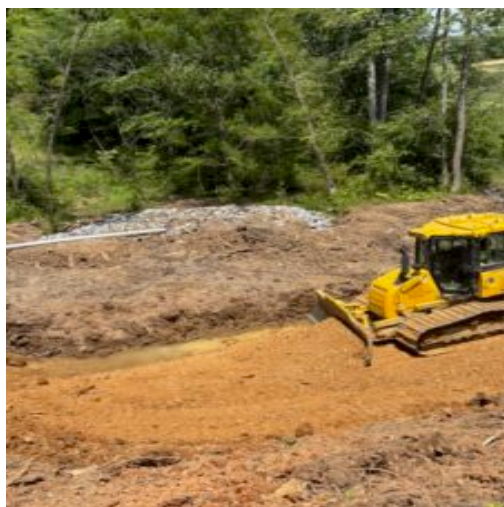
Spreading fill using dozer
