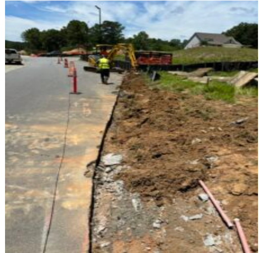
Removing curbing at round about
