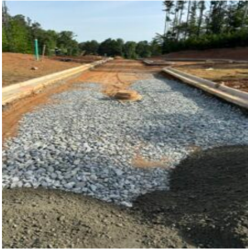
#34 stone placed at repaired sub grade
