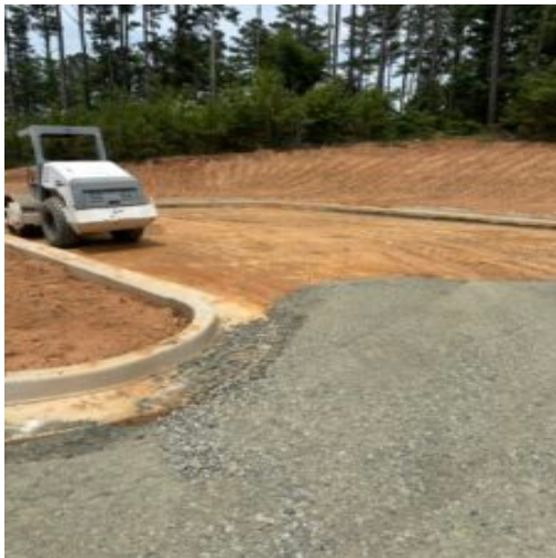
Placing base stone(GAB) over repaired sub grade
