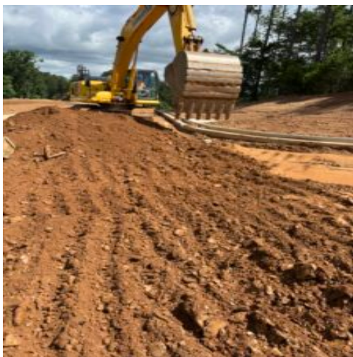
Undercutting and clipping existing saturated sub grade soils -8" to -6", observing by probing using a rounded end steel rod.
