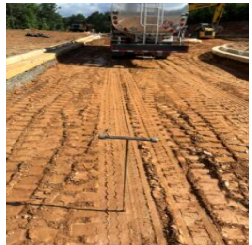
Undercutting and clipping existing saturated sub grade soils -8" to -6", observing by probing using a rounded end steel rod.
