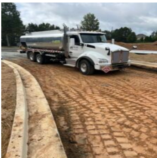
Fuel truck observed on sub grade with no movement after clipping.
