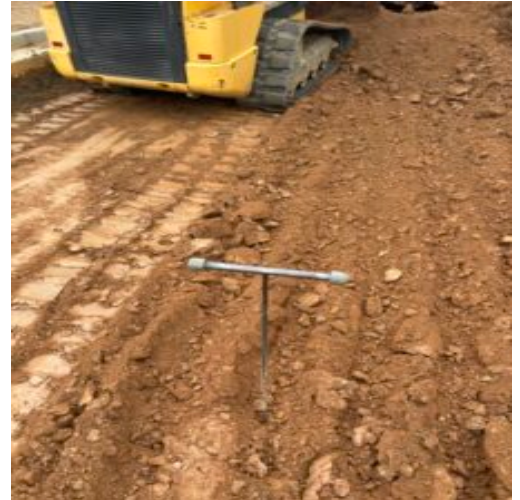
Probing using a rounded end steel rod
