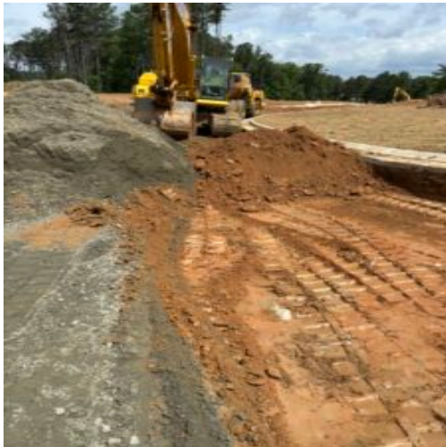
Sub grade clipped -6" at entrance drive
