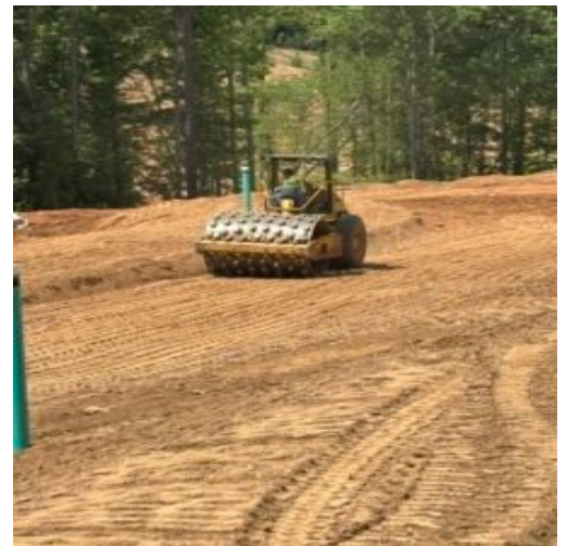
Compacting between #10 and 11
