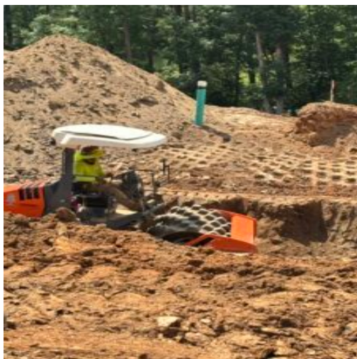
Compacting fill at sanitary sewer line between manhole # 11 and 12
