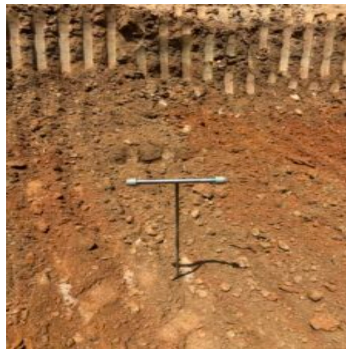
Undercut area at lot # 27
