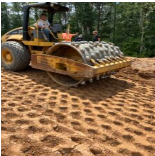
Compacting undercut area at lot #27
