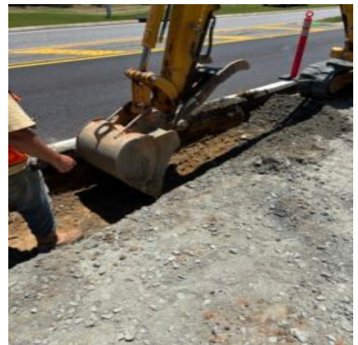
Observing subgrade after removal of existing curb at Seven Hills
