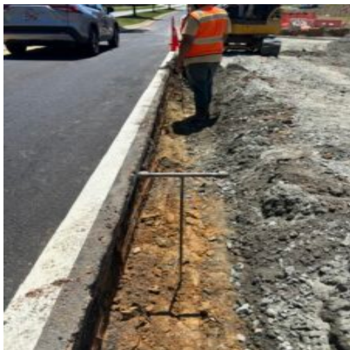
Observing subgrade after removal of existing curb at Seven Hills
