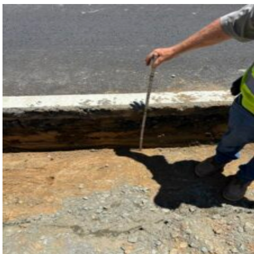
Observing subgrade after removal of existing curb at Seven Hills
