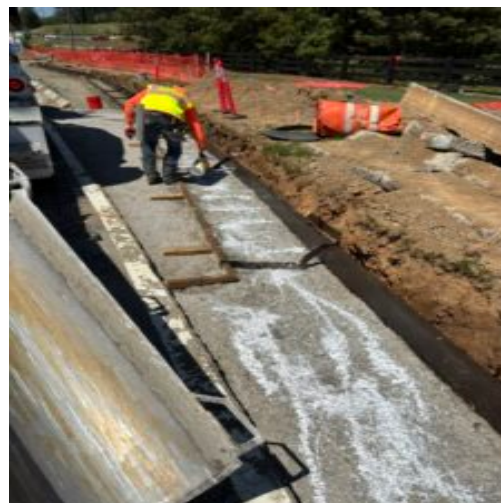
Bonding agent poured previous poured concrete
