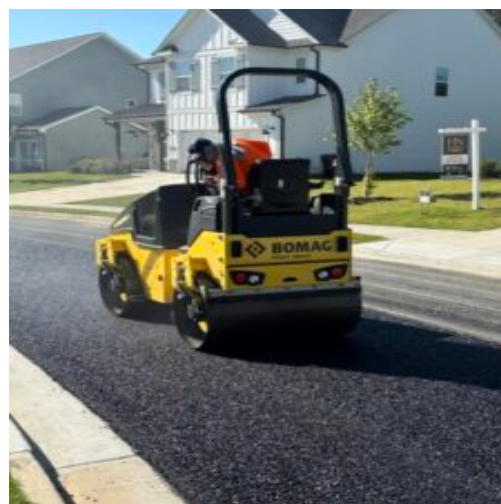
Compacting Perma Pave
