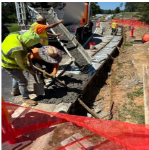
Curbing poured at tapered end after bonding agent was poured over previous concrete pour
