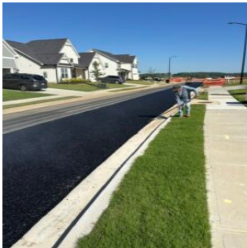
Perma Pavement placement
