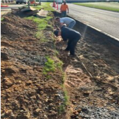
Removal of saturated silt at tapered end
