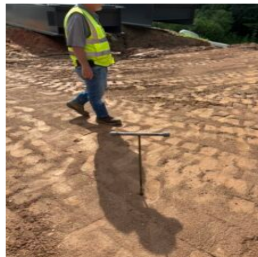
Sub grade observation at bridge approach crane pad using probe rod
