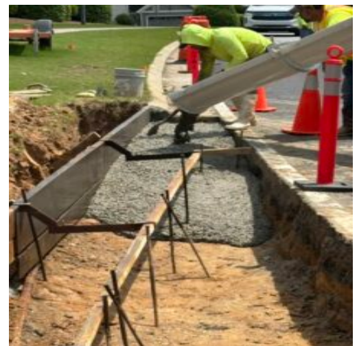
Class B concrete pour at tapered end decel lane using a 4000 psi mix at Seven Hills Boulevard .
