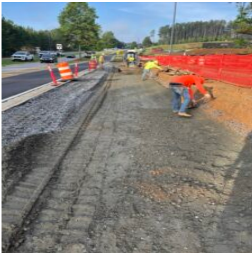
Removal of saturated silt at tapered end
