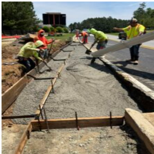
Class B concrete pour at tapered end decel lane using a 4000 psi mix at Seven Hills Boulevard .
