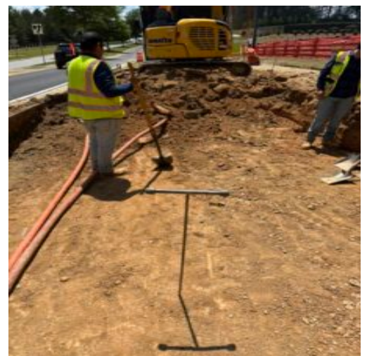
Excavated subgrades at deceleration lane showing observation by probing with utilities in place. Also showing depth excavated of 25" from top of curb.
