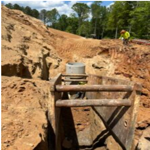
Installation of 8" ductile iron sewer line
